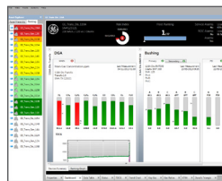
Transformer health/risk overview
